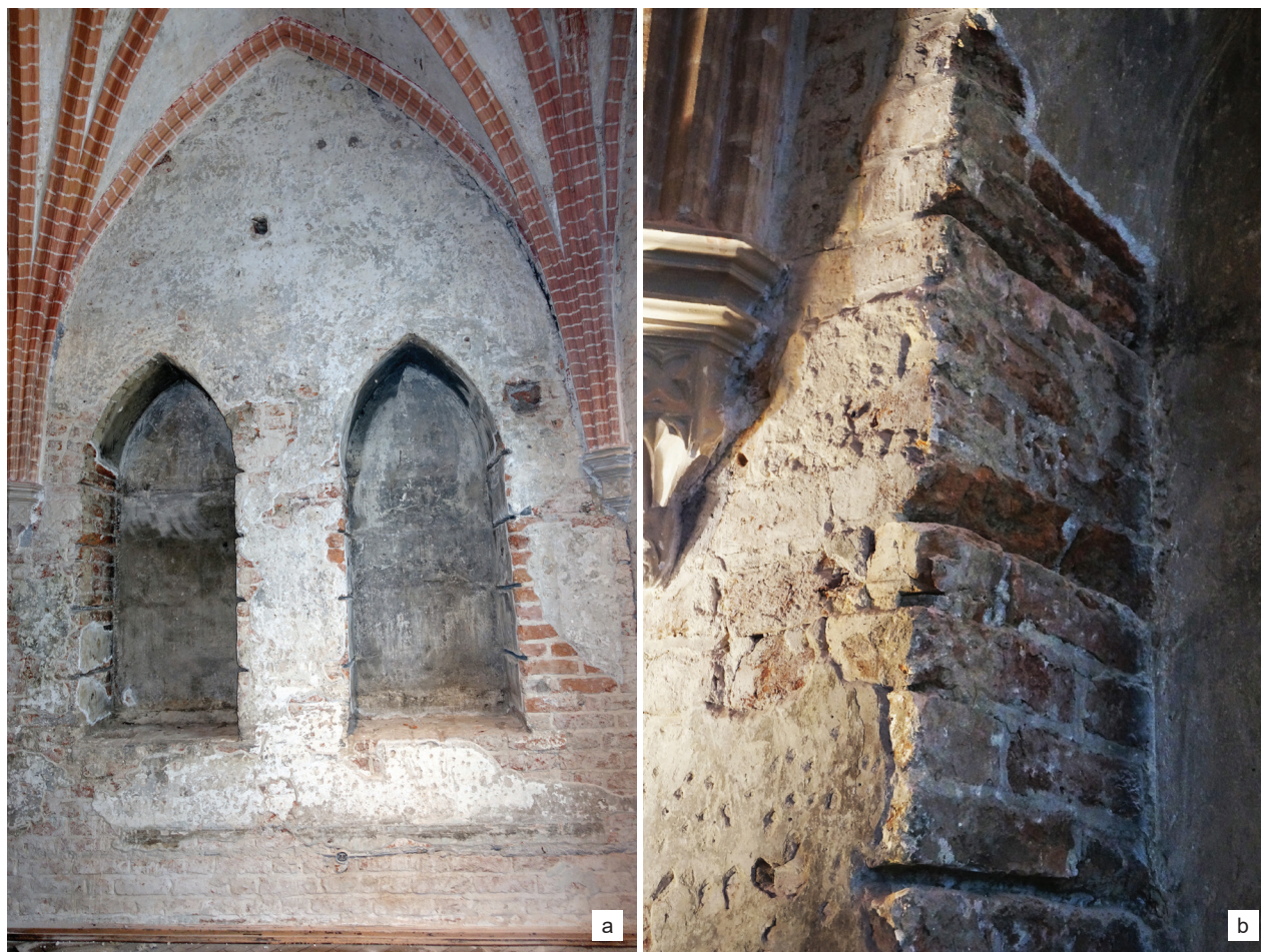
Fig. 5. The northern bay of the western wall with a pair of ogival recesses. Their side walls contain horizontally bevelled and right-angled cuts so that shelves could be fitted: a) general view, b) detail with cuts in the southern wall of the second recess from the north (photo by A. Piwek)
