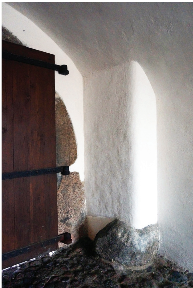
Fig. 7. The eastern fragment of the medieval entrance to the Kwidzyn castle with a late-Gothic extension (pilaster) and a modern segmental vault (photo by A. Piwek)
