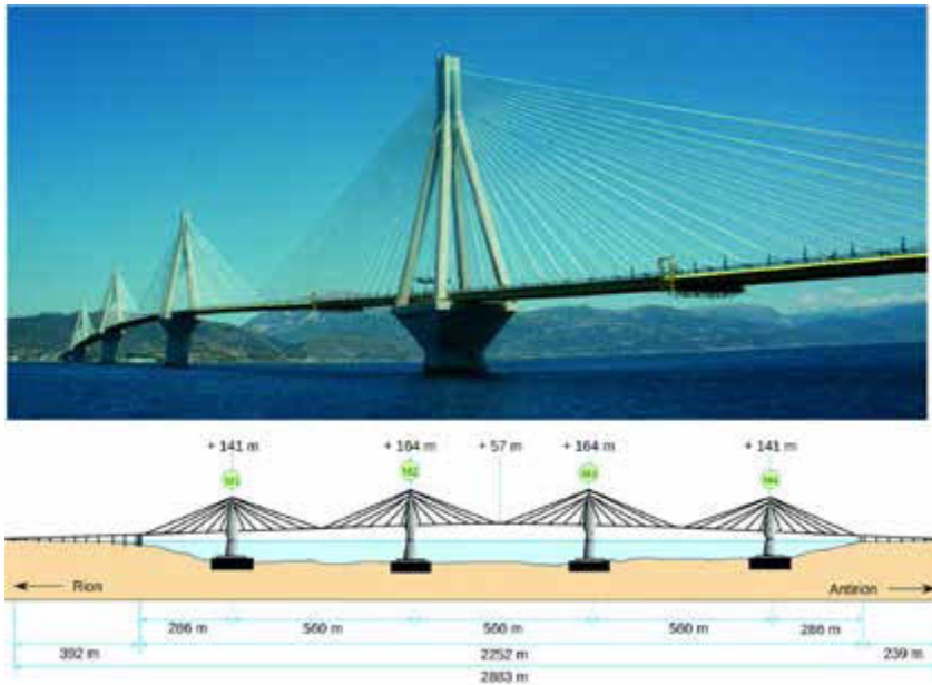
Fig. 41. Rion-Antirion Bridge. Greece, Jacques Combault, 2004 [5], (photo: wikipedia.com)
