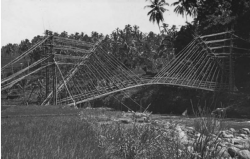
Fig. 1. Bridge constructed of bamboo, Java, 1930 (photo: digitalcommons.brockport.edu)
