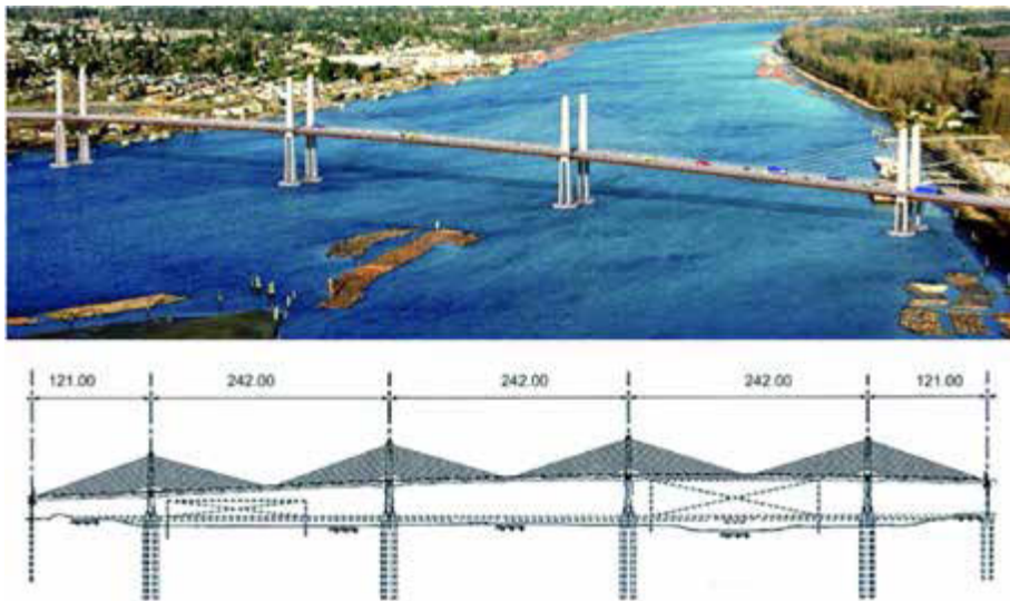
Fig. 37. Golden Ears Bridge, Vancouver, Canada, Miller Group 2009, [5], (fot. The Miller Group)
