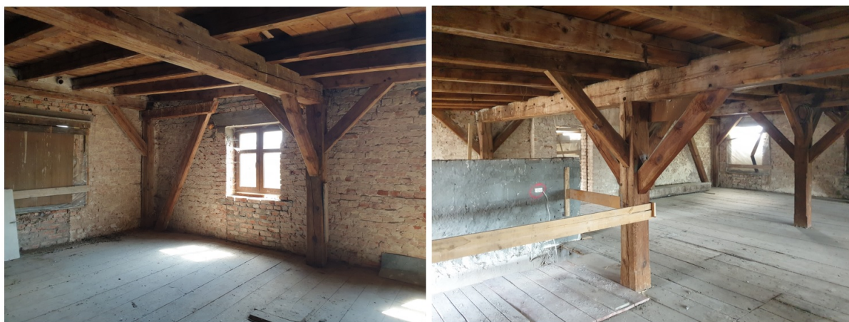
Figure 1. Example of the use of wood in the construction of a ceiling.
