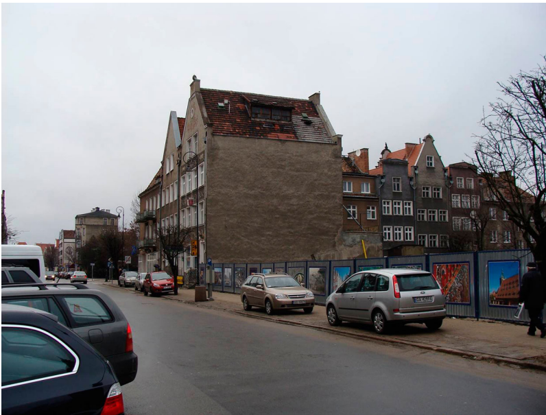
Figure 3. View of the site before the construction of the block. Source: photo by A. Taraszkiewicz, 2010
