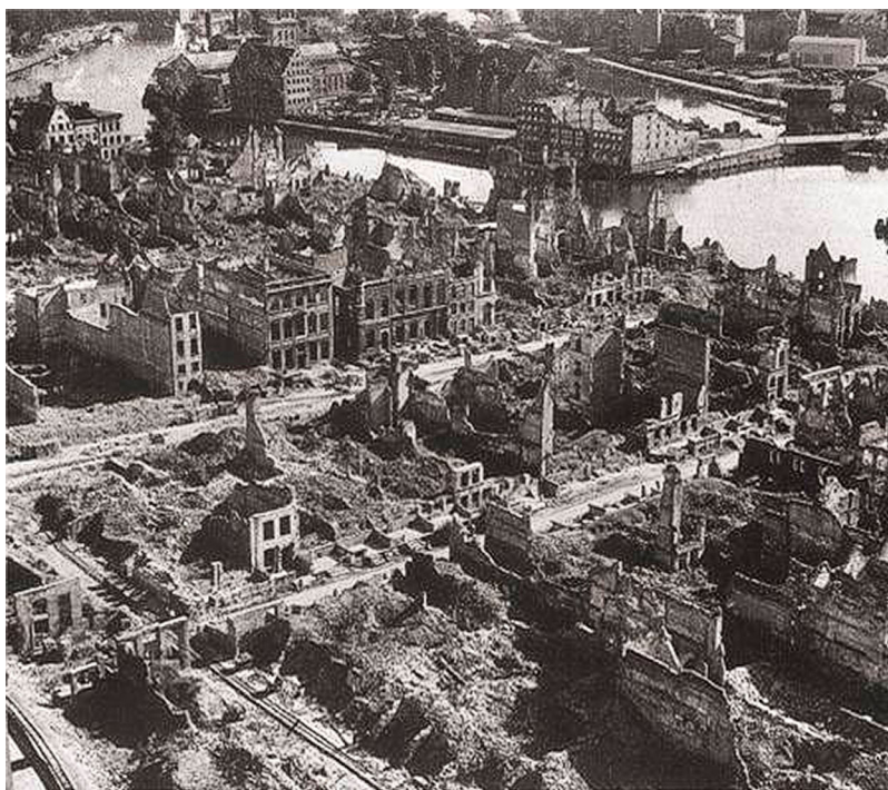
Figure 1. Photograph of damage in Gdańsk after the Second World War. Source: (Cieślak and Biernat 1994)
