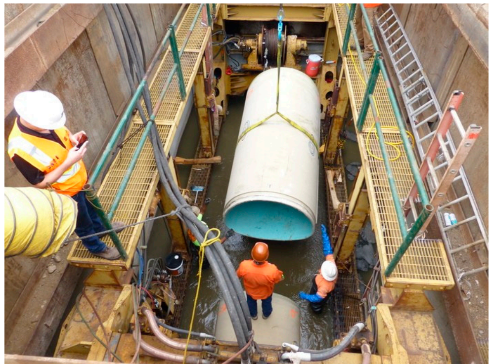
Figure 18. Aligning the segment with the host pipe [34].
