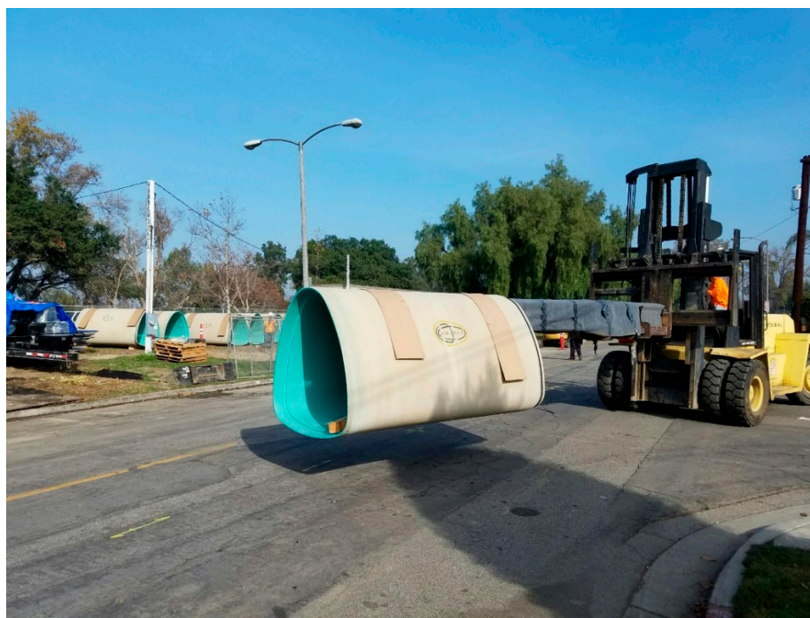
Figure 15. Unloading and transportation of segments of pipe on-site [34].
