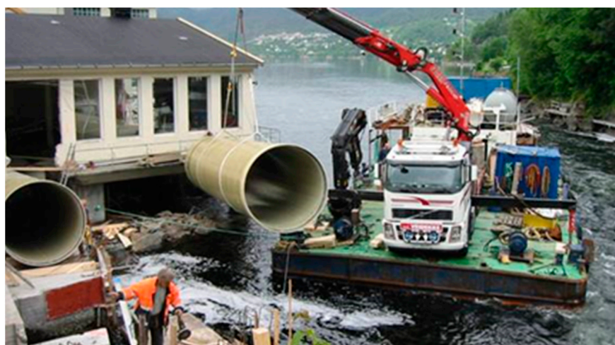
Figure 14. Installation of pipes from barge [18].
