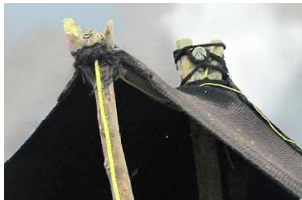
Fig. 127: Soleimani Tribe. columns with a groove/forked end and placement of horizontal beams on them, photo by author
