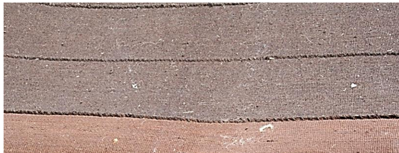
Fig. 95: Narrow strips of Black Tent roof cover are sewn together and while on the roof, the seams are parallel to the ridge of the roof ;Qashqai Tribe, Fars Province, photo by author
