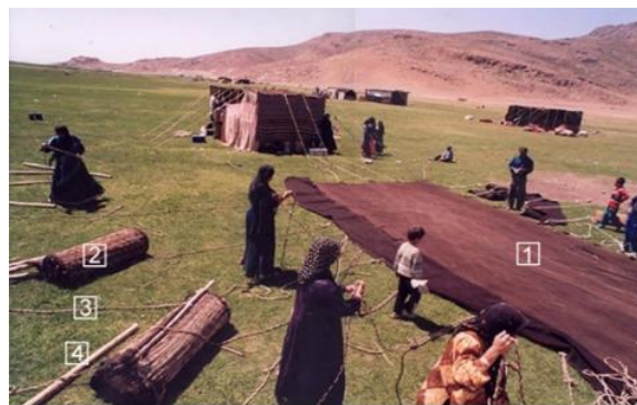
1. Tent fabric (Roof) 2. Alachigh 3. Rope 4. Post
