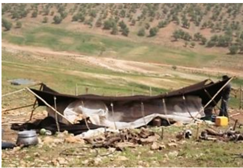
Fig. 76: Slanting position of corner columns Photo by author
