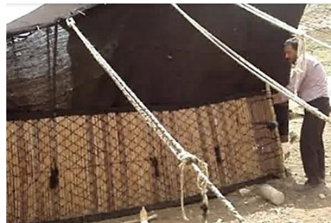
Fig. 87: Thin branches are rammed/pounded into the ground and Chigh is unwind to support the wall, photo by author
