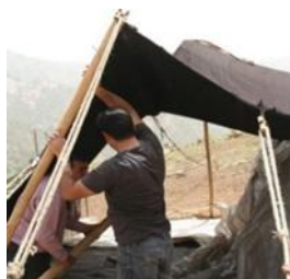
Fig. 79: Pulling up the end and the middle column which carries a ridge beam, photo.
