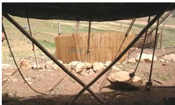
Fig. 83: The posts are arranged along the walls of the tent in a criss-crossed way (bracings), photo by author
