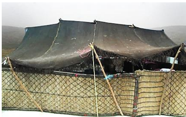
Fig. 124: Soleimani Tribe. Four parts of the tent's roof cover are joined by the metal pins, photo by author
