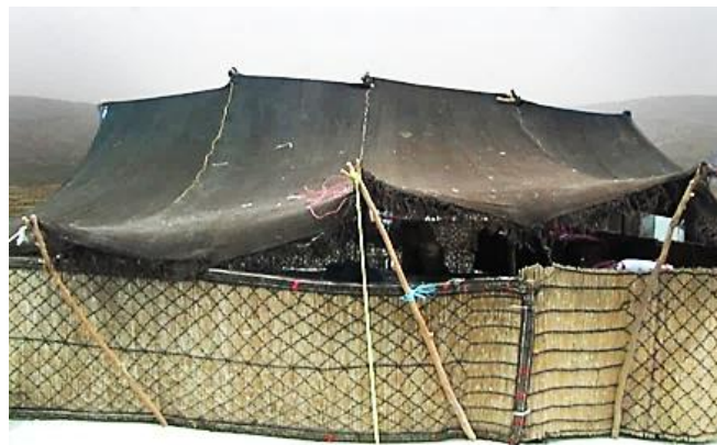
Fig. 124: Soleimani Tribe. Four parts of the tent's roof cover are joined by the metal pins, photo by author
