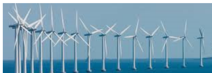
Figure 12. Wind turbine farm [82].
