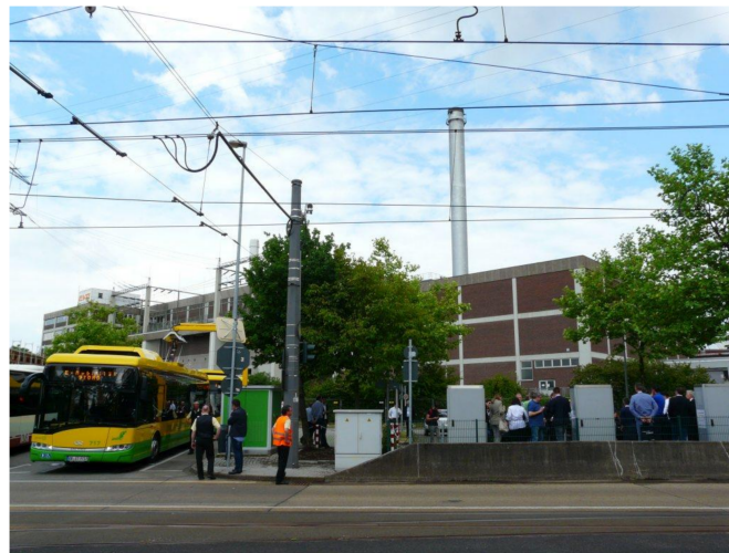
Figure 3. Charging station for electric bus and electric cars powered from the tram overhead line in Oberhausen, Germany.
