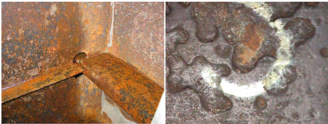
Figure 1. The comparison between general (left) and pitting (right) corrosion (International Association of Classification Societies, 2015).
