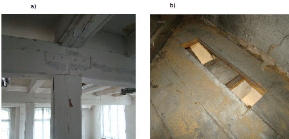
Figure 9. Building planned for modernization - ceiling above the second floor: a) a fragment of a wooden frame, b) a structure of the ceiling
