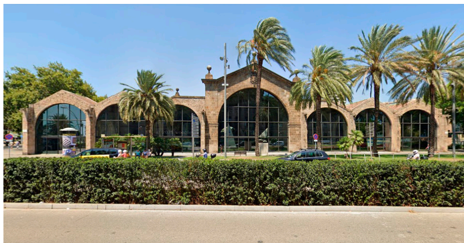
Figure 8. An example application of a laminated glass wall on a historic building of the Maritime Museum of the Barcelona Shipyard from the Medieval period—January 2022.
