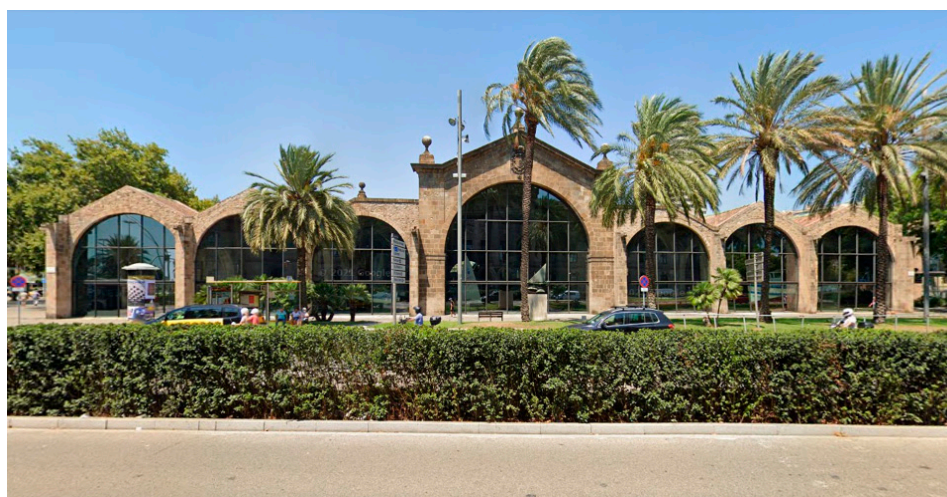
Figure 8. An example application of a laminated glass wall on a historic building of the Maritime Museum of the Barcelona Shipyard from the Medieval period—January 2022.
