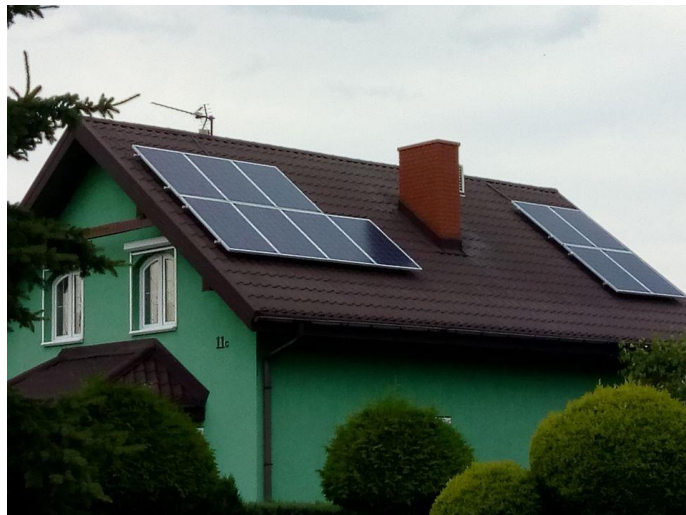
Fig. 2. A private investor's roof PV system, Lubień Kujawski, Poland (photo: B. Igliński)
