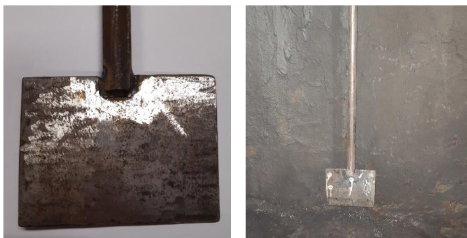
Figure 14. View of the reference plate installed inside the classifier tank.
