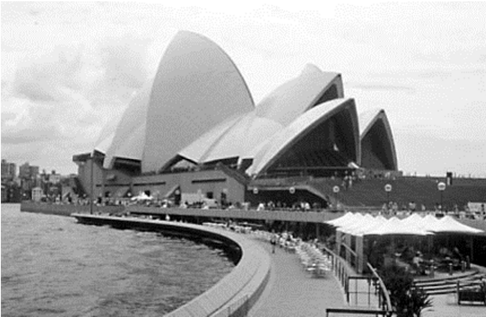
Figure 2. Exterior View of the Sydney Opera House.
