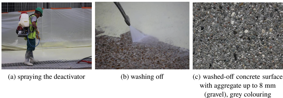
Fig. 1. The technology of processing the surface by means of using a retarding agent
