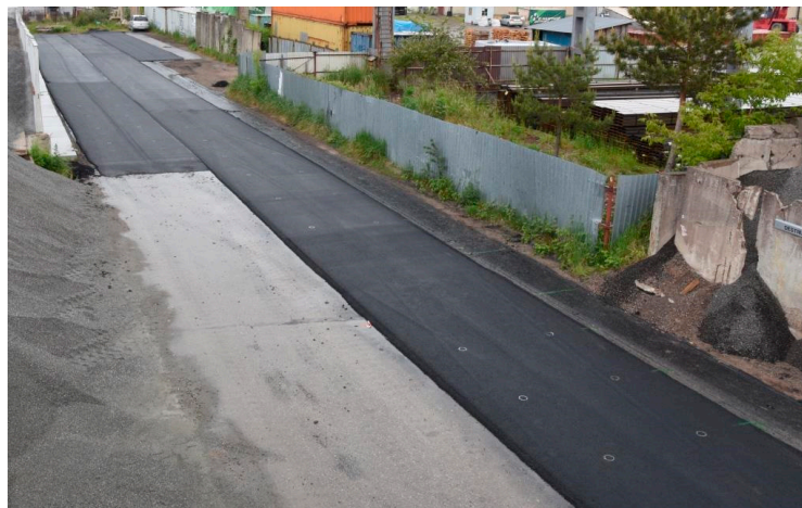
Figure 11. Second short test section located at the asphalt plant (MTM2)—June 2020.
