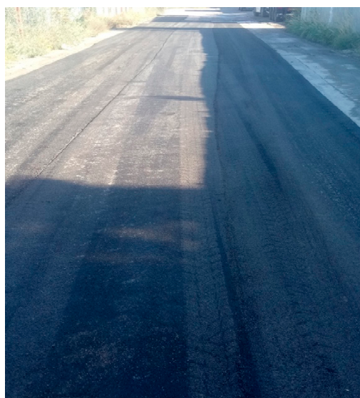
Figure 8. First short test section at the asphalt plant (MTM1) constructed during technological trials described in Section 3.6—September 2018.
