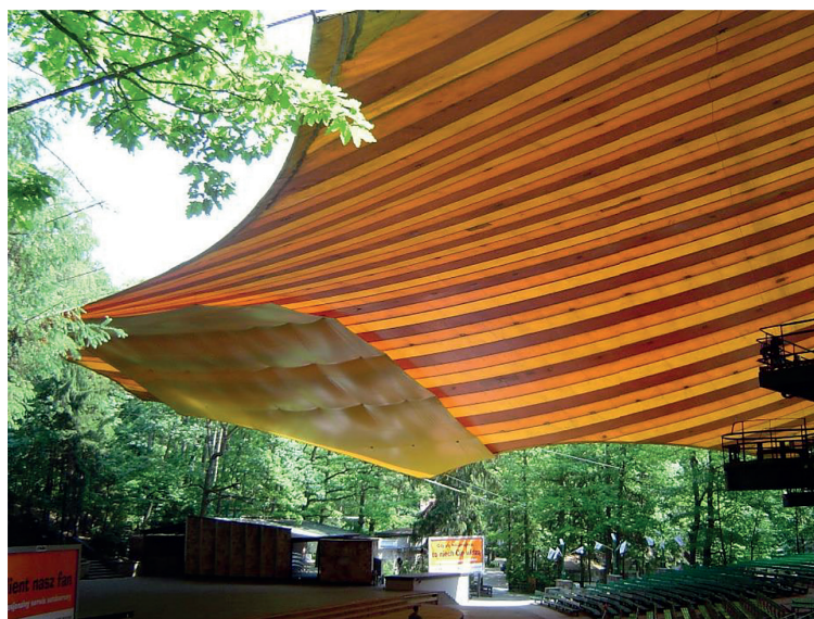
Fig. 3. Roof of the Forest Opera in Sopot (2009).
