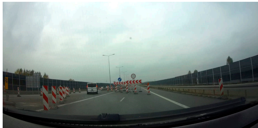
Figure 5. Example of a recorded event—unexpected road works.
