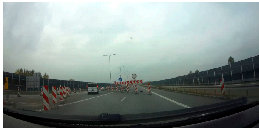
Figure 5. Example of a recorded event—unexpected road works.
