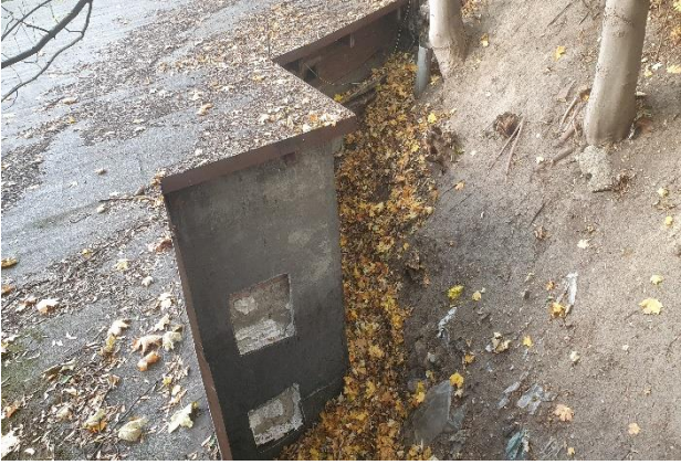
Photo. 4: Steps of the external wall (from the escarpment side) of the former office rooms (A)
