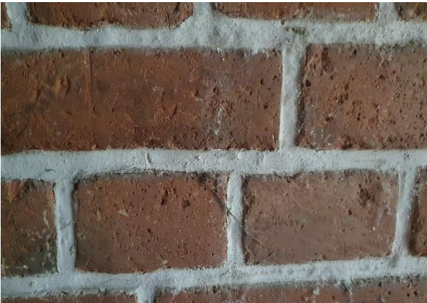
Photo. 6: Salting the walls inside the rooms of the former service apartment (B)
