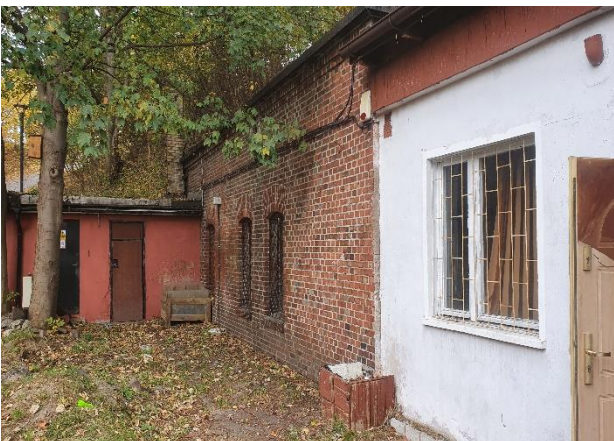
Photo. 3: Utility rooms (C) adjacent to the former service apartment (B)
