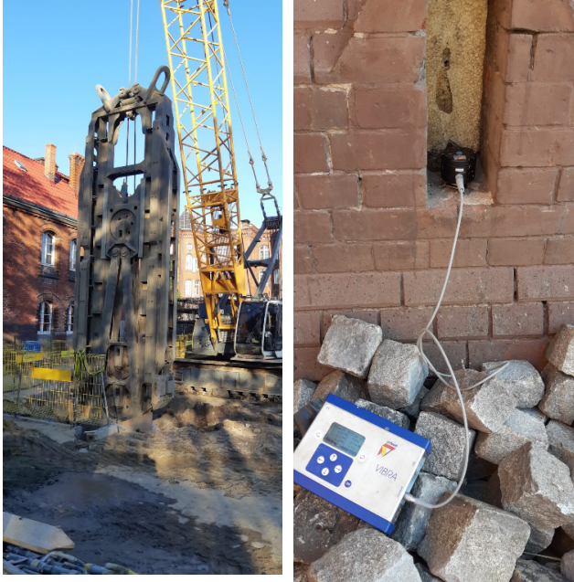
Figure 4: The examined case: structure sensitive to dynamic excitation located in the vicinity of diaphragm wall installation (a); vibration monitoring made on structure (b).
