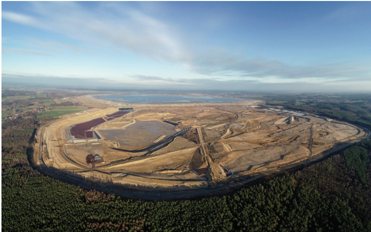
Fig. 1. The Żelazny Most tailings storage facility (OUOW) with the South Headquaters under construction – the main building of the Hydrotechnical Department
