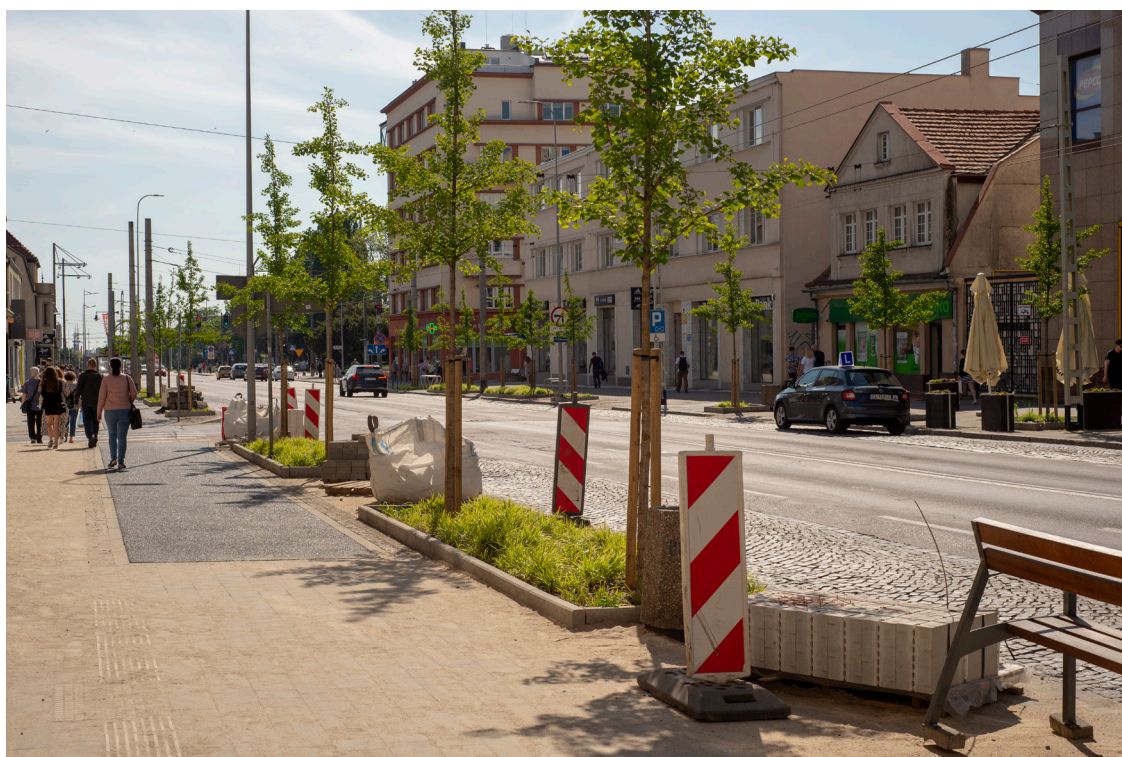
Fig. 3. Gdynia, 10 Lutego Street, after renovation works, which included the conversion of parking bays as well as the reintroduction of the historic width of pavements and the replanting of trees; photo by B. Ponikiewski.
