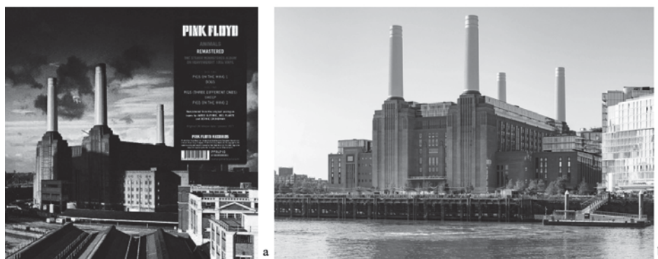
Figure 10 a,b. Battersea Power Station as a popularized Industrial Icon & its 2022 renewal.
