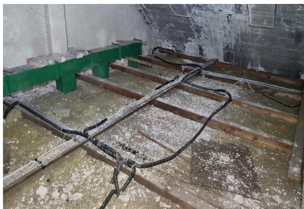
Photo 7. Warehouse building - attic space: a) arrangement of wooden ceiling beams of the covering structure above the ground floor, b) supporting wooden ceiling beams on a horizontal tie
