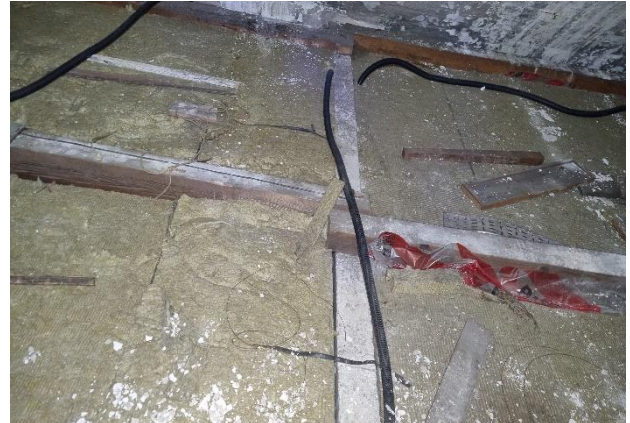
Photo 7. Warehouse building - attic space: a) arrangement of wooden ceiling beams of the covering structure above the ground floor, b) supporting wooden ceiling beams on a horizontal tie
