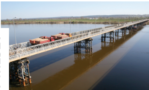
Figure 3. DMS-65 detour bridge, Chełmno, Poland
