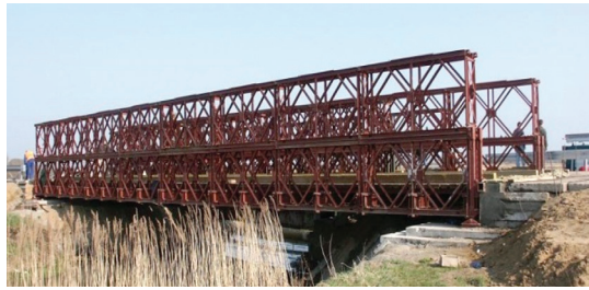
Figure 2. Diversion road with MS 22-80 bridge
