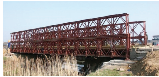
Figure 2. Diversion road with MS 22-80 bridge
