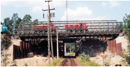
Figure 2. Diversion road with MS 22-80 bridge
