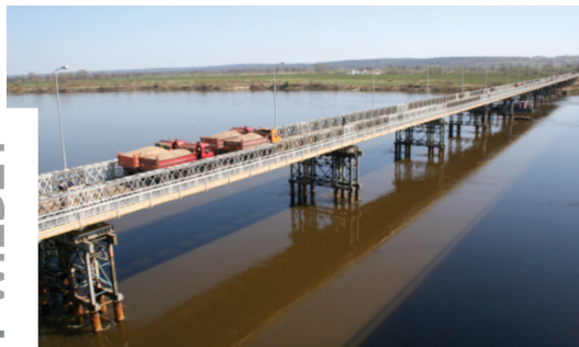
Figure 3. DMS-65 detour bridge, Chełmno, Poland
