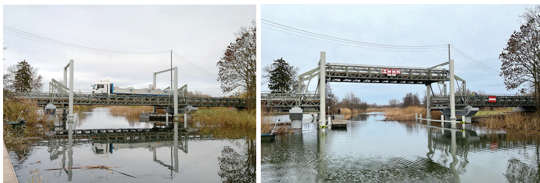
Figure 13. Views on the bridge over the Tuga River in Żelichowo, Poland: A road and sailing serviceability stage
