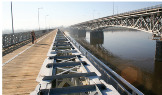
Figure 3. DMS-65 detour bridge, Chełmno, Poland
