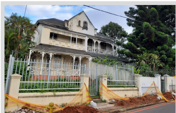
Figure 4-13 - 76/78 Hunt Rd. This 'Colonial' duplex has two units, each over two floors. In this particular instance, one unit is classified as being in a 'poor condition' as it requires a considerable amount of maintenance and this impacts on the overall building. The property ownership is usually separate for this period of construction, so it is difficult for the owner of the adjoining unit to practically influence ongoing maintenance. The formation of Sectional Title ownership addresses this shortcoming to a significant extent, though interpersonal relationships work better when there are larger numbers of owners that make up the sectional title.
