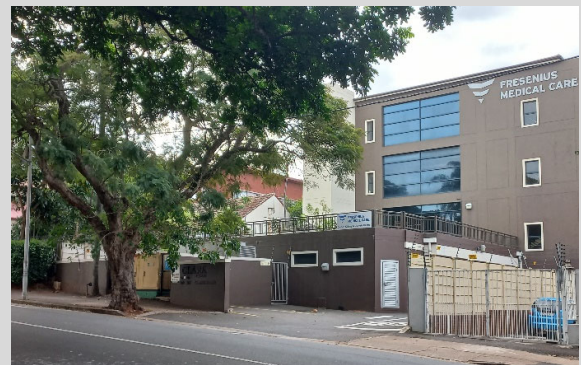
Figure 5-25 - Clark Square (260/262 Clark Rd.) This site would have originally been a single dwelling house that has been demolished and has been replaced by this medical centre. This has a municipal substation on the boundary (seen behind the tree trunk) in addition to a electrical switch room (located behind the solid metal door to the right thereof). The entire focus of the street frontage at road level is on servicing, though the building behind it is not particularly complementary to the streetscape either.
