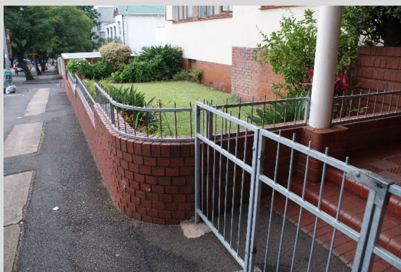
Figure 5-31 - Wyndham (408 Che Guevara Rd.) The low face brick wall defining the property boundary had subsequent addition of low steel panels and fence, more to stop the use of them as seats. Unfortunately, since the taking of this photograph, a higher fence has been erected.
