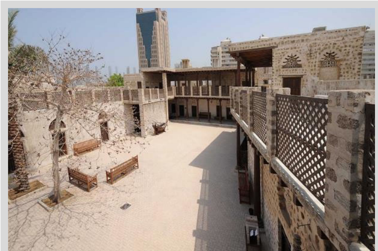
Figure 3-3 – The Beit el-Nabudah Sharjah restoration project follows more traditional conservation techniques within the urban realm, which in turn helps to activate further interventions towards creating a suitable urban historical identity. Source: (Heart of Sharjah, 2016)
