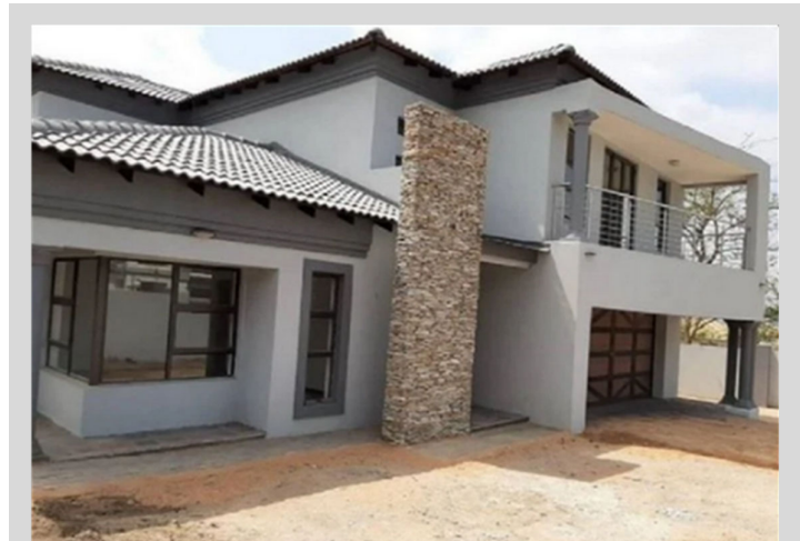
Figure 2-51 - The "most famous house in South Africa" on the 18th February 2020. This was a viral Twitter topic during the preceding days. Located in the Drum Rock lifestyle estate in Nelspruit, Mpumalanga province, this faux Tuscan development is indicative of an inappropriate developer driven language being marketed as the 'ideal home' and unfortunately seen as such by a significant number of individuals. Source: (Caboz, 2020)
