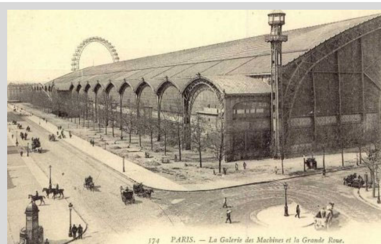
Figure 3-8 - Ferdinand Dutert's Palais des machines (1889), the largest vaulted building to have been built at its time of construction is another later example of the pragmatism of engineering being the primary design driver. Source: (Wikimedia Commons, 2016)
