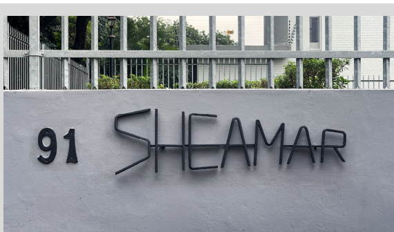
Figure 5-53 - Sheamar (91 Lena Ahrens Rd.) Here shaped metal flat bar has been used to form the building signage. The building number is an 'off the shelf' standard hardware store item undoubtedly added some time later.
