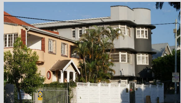
Figure 5-46 – Ashburn (358 Che Guevara Rd.) A common detail with modernist apartment buildings is to have a parapet wall facing the street and a pitched roof behind the parapet. This presents the horizontal line between building and sky synonymous with international modernist ideals while incorporating the practicality of a sheeted inclined roof in the local construction context.
