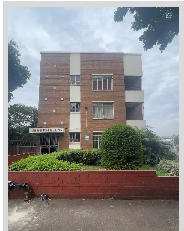
Figure 5-48 - Markhall (45 Lena Ahrens Rd.) The use of varying panels of face brick and plaster adds variety to the façade articulation. This can be used to superficially create panels in a uniform volume (such as the plaster strip to the left) or to define volumes (such as the balcony elements, finished in plaster, on the right).
