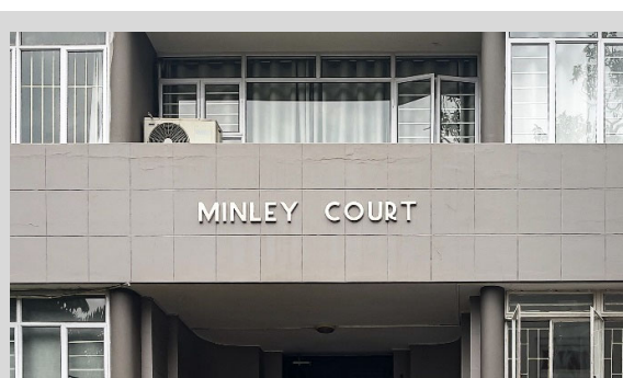
Figure 5-55 - Minley Court (138 Lena Ahrens Rd.) The use of pre-formed lettering affixed to a wall or on top of a slab projection above the entrance is a very common element in mid-century modern apartment buildings. The lettering type (font) is also fairly consistent, with a very limited number of exceptions.
