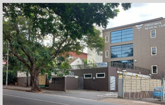
Figure 5-25 - Clark Square (260/262 Clark Rd.) This site would have originally been a single dwelling house that has been demolished and has been replaced by this medical centre. This has a municipal substation on the boundary (seen behind the tree trunk) in addition to a electrical switch room (located behind the solid metal door to the right thereof). The entire focus of the street frontage at road level is on servicing, though the building behind it is not particularly complementary to the streetscape either.
