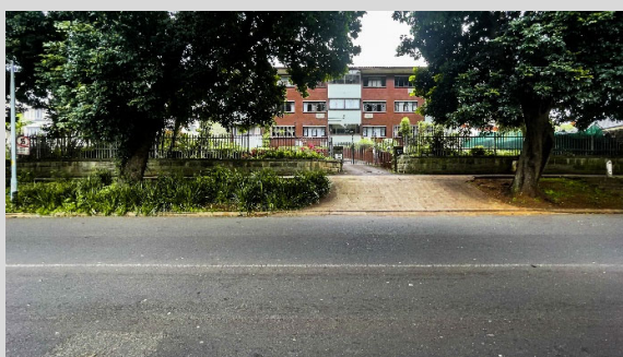
Figure 5-30 - Lincoln Hall (92 Lena Ahrens Rd.) This forms part of the Lena Ahrens Rd section that has noted landscaping along the pavement. The pavement is raised in relation to the road and the embankment between is planted. Though the maintenance of this is for the local authority, many property owners take responsibility due to the lack of capacity demonstrated by the local authority.
