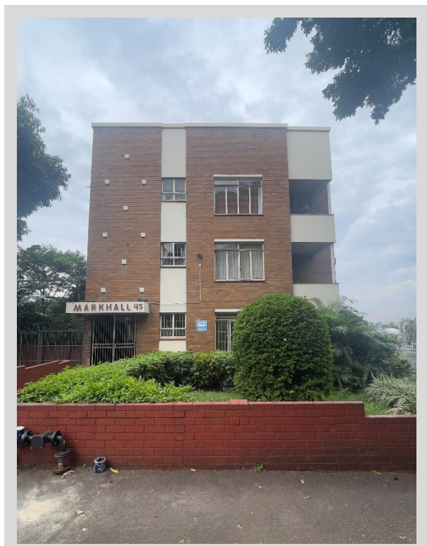
Figure 5-48 - Markhall (45 Lena Ahrens Rd.) The use of varying panels of face brick and plaster adds variety to the façade articulation. This can be used to superficially create panels in a uniform volume (such as the plaster strip to the left) or to define volumes (such as the balcony elements, finished in plaster, on the right).
