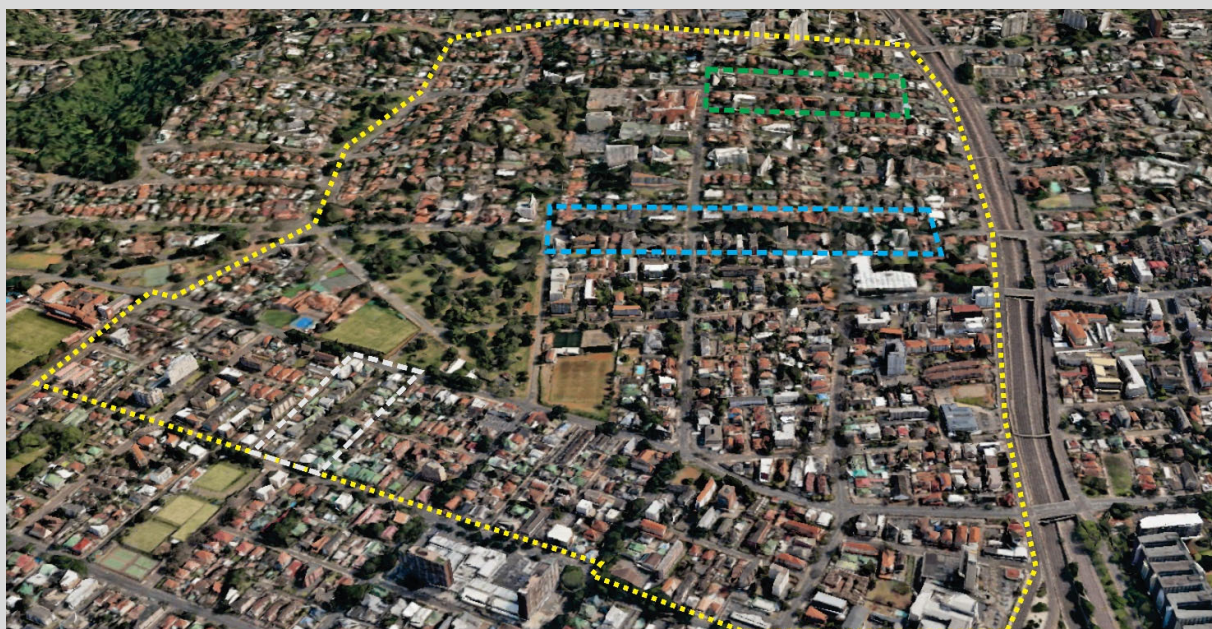
Figure 5-19 - Aerial overview of the study area. The yellow outline of the study area boundary, the grey outline is the Ferguson Road detailed survey node, the blue outline is the Lena Ahrens detailed survey node, and the green outline is the J.B. Marks detailed survey node. Source: (Google Earth, 2015(a))
