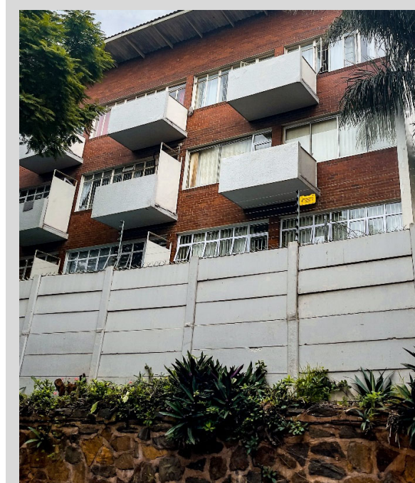
Figure 5-42 – Camberly Hall (134 Lena Ahrens Rd.) The balconies are expressed as a series of ‘prominently projecting ‘clipped on’ masses, adding dynamism to what would otherwise be a rather bland elevation.
