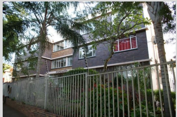
Figure 2-55 - Moorehaven, 1948, 375 Che Guevara Rd. The rather familiar sight of the subsequently added fencing of palisade and electric capping to the original low garden boundary wall. The visual flow is definitely compromised, but there is still some measure of transparency.
