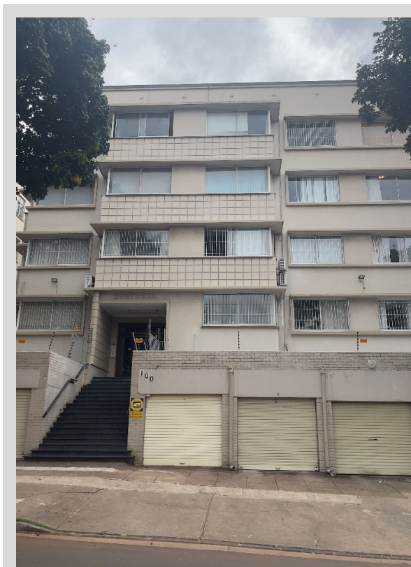
Figure 5-58 – Montreal (100 J.B. Marks Rd.) The entrance here is placed off centre in a centrally defined volume, though entry is made unmistakable by the prominent stairs leading from the pavement in the only gap between garages that line the entire property boundary.
