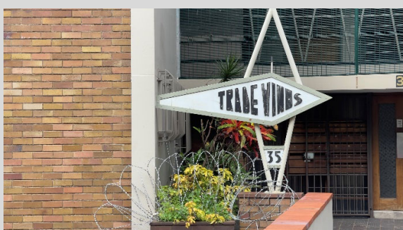
Figure 5-54 - Trade Winds (35 Lena Ahrens Rd.) This is one of the most elaborate and considered building signage in the study area. Cut out letters are affixed to a plane contained in a custom steel frame. This unfortunately is now fairly removed from the public sphere are additional due to the erecting of a boundary fence and gate.
