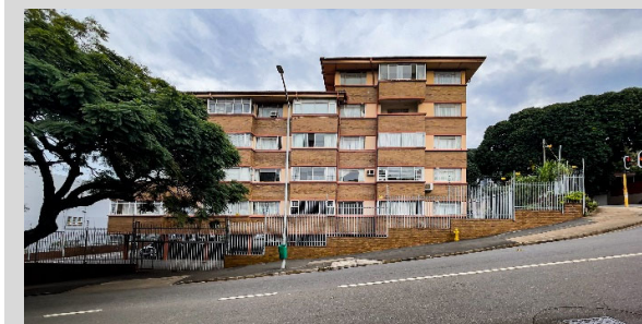
Figure 5-24 – Brierly (55 J.B. Marks Rd.) demonstrates the advantageous use of the slope. Entrance is around the corner from the top of the slope by means of a bridge, therefore an entire floor of accommodation and parking can be incorporated without exceeding the four storey height constraint.
