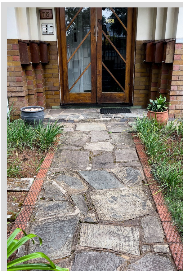
Figure 5-35 - Wilfton (75 Ferguson Rd.) The slasto garden path with clay brick border echoes the use of 'natural materials' along with the face brick plinth and timber framed entrance doors.
