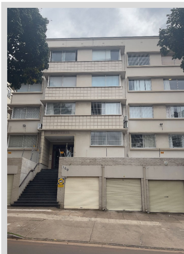
Figure 5-58 – Montreal (100 J.B. Marks Rd.) The entrance here is placed off centre in a centrally defined volume, though entry is made unmistakable by the prominent stairs leading from the pavement in the only gap between garages that line the entire property boundary.
