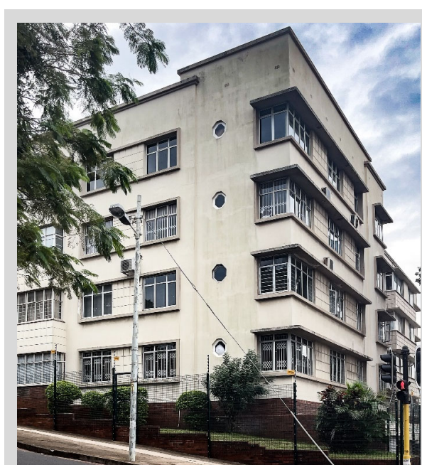
Figure 5-27 - Mount Verna (104 J.B. Marks Rd.) This is one of the examples of all of the corner plot buildings in the J.B. Marks node addressing both street edges.
