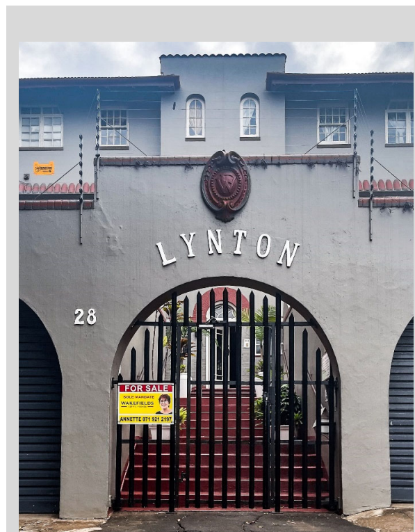
Figure 5-59 - Lynton (28 Lena Ahrens Rd.) Though somewhat obscured by the boundary treatment (which may be subsequent to the original construction), the entrance definition is enhanced by the use of an extension to the parapet wall above it in addition to the overall volume containing it sitting slightly proud to its surrounds.
