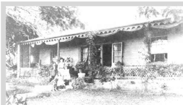
Figure 2-19 - 'Longlands' (c. 1875) is an example of the typical homes first built on the Berea. The brick and iron roofed structure with vertically proportioned windows and wrap around verandah. The canvas awnings would later translate into the bracket profiles included on later houses. Source: (Kearney, 1984)
