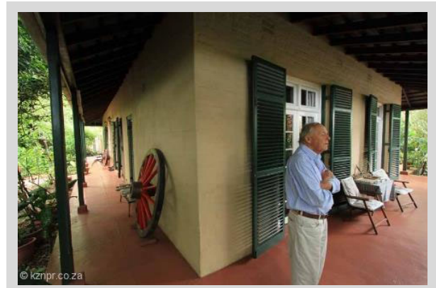
Figure 2-20 - Recent image of the restored Elephant House. The long, narrow building with wrap around verandahs typifies the earliest buildings on the Berea, such as 'Longlands'. Source: (Bland, H, 2020)
