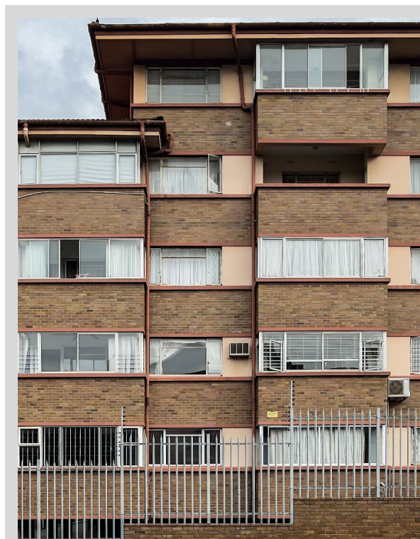
Figure 5-63 - Brierly (55 J.B. Marks Rd.). In this image only one of the balconies remain as original and unenclosed. The use of sliding windows is almost universally only found in these subsequent balcony enclosures. There is no uniformity of detailing in the enclosing, which negatively affects the perception of the visual quality.
