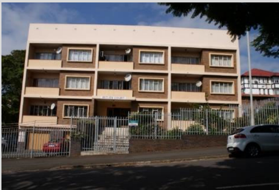
Figure 2-54 - Witley Court, 1953, 510 Che Guevara Rd. The building demonstrates the tendency of the time to have balconies and large openings facing the street. The palisade fencing is a recent addition.
