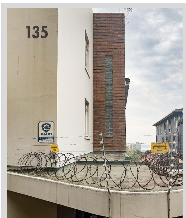
Figure 5-62 - Glenalvon (135 Lena Ahrens Road). Though rather prominent in the image is the rusting barbed wire, the image also highlights the restrained use of glass bricks in a face brick defined volume. It is practical in that it lets light into the stairwell where windows would otherwise be difficult to access and clean. The varied, yet restrained use of materials with natural appearance includes the slasto covering to the path and the sandstone cladding to the right of the entrance door.
