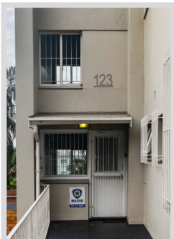
Figure 5-39 - Manning Hall (123 Lena Ahrens Rd.) Many examples exist across the study area where an additional security gate has been added to the original main building entrance door.
