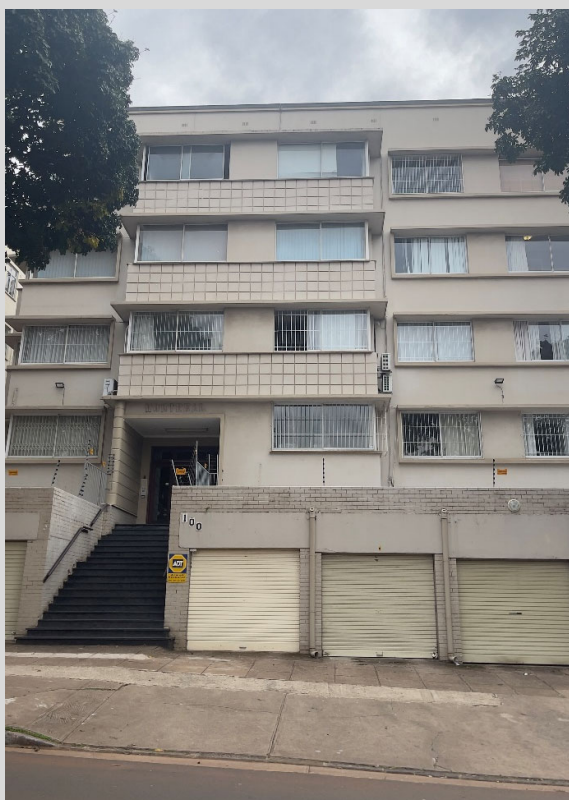
Figure 5-58 – Montreal (100 J.B. Marks Rd.) The entrance here is placed off centre in a centrally defined volume, though entry is made unmistakable by the prominent stairs leading from the pavement in the only gap between garages that line the entire property boundary.
