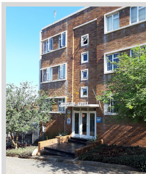
Figure 5-38 - Magister Court (11 Muthaiga Place). Though just beyond the study area, this is an example of security adaptations that try to retain the original streetscape character. Fencing is at the side of the building in line with the front façade and the additional entrance security gate is within the entrance lobby. Barely visible in this image, it also uses electric fencing in the façade, running just beneath the ground floor window cills and over the top of the entrance slab.
