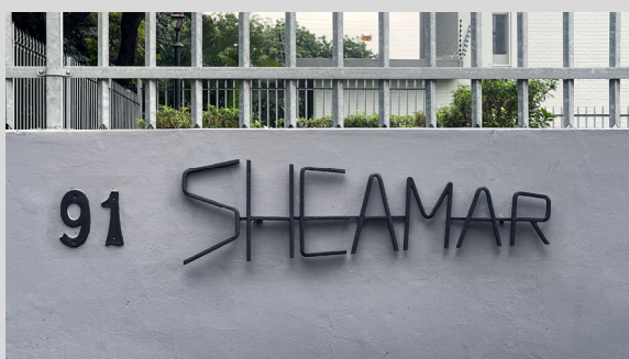
Figure 5-53 - Sheamar (91 Lena Ahrens Rd.) Here shaped metal flat bar has been used to form the building signage. The building number is an 'off the shelf' standard hardware store item undoubtedly added some time later.
