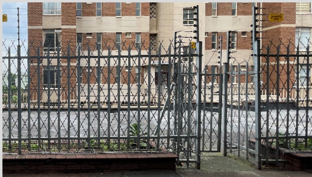
Figure 5-37 - Strelitzia (81 Lena Ahrens Rd.) The original low planter boxes along the boundary now have this rather intimidating boundary fencing setup – Palisade fencing with razor mech panels and electric fencing on top. This reinforces the notion of an unsafe street.
