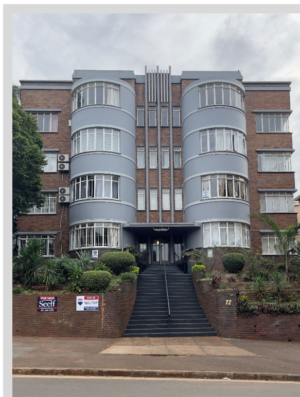
Figure 5-44 - Algwen (72 J.B. Marks Rd.) The elevation demonstrates what this study terms ‘major visual density’, though this is relative to the study area context. The combination of vertical and horizontal lines, intersecting semi-circular volumes with a rectangular one and panels in varying relief to one another are well considered and composed here. The overall façade treatment is complex without being uncontrolled.
