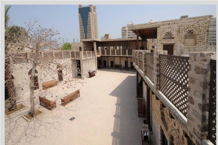
Figure 3-3 – The Beit el-Nabudah Sharjah restoration project follows more traditional conservation techniques within the urban realm, which in turn helps to activate further interventions towards creating a suitable urban historical identity. Source: (Heart of Sharjah, 2016)
