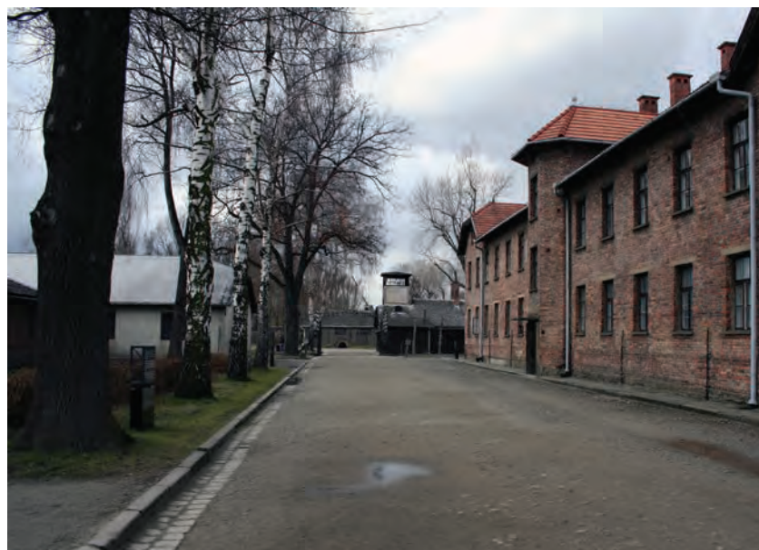
2. The internal road leading from the main gate
