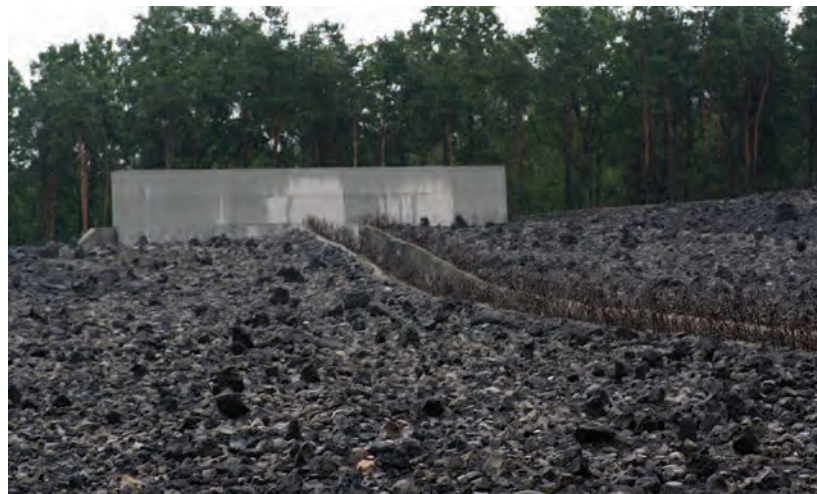
4. The hill cut by the crevasse
