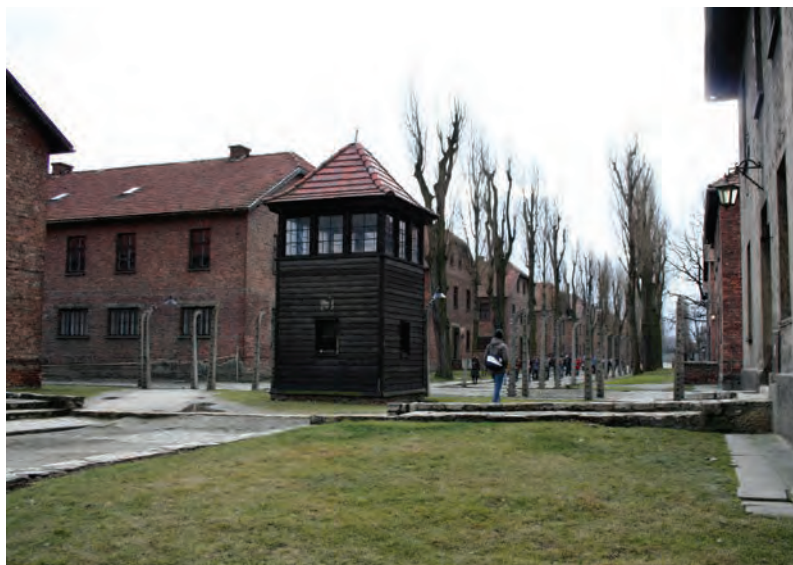
4. The internal road between the prisoner blocks
