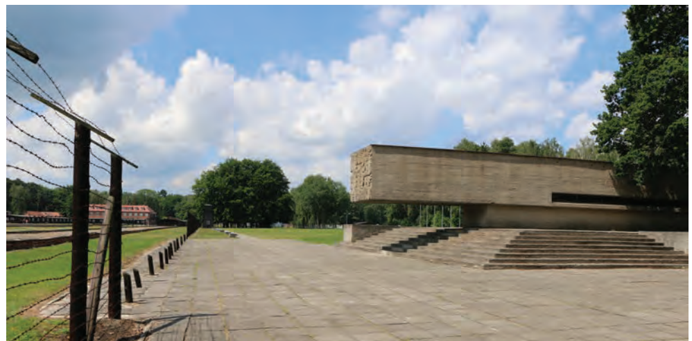
8. The symbolic overhanging of the horizontal part of the monument
