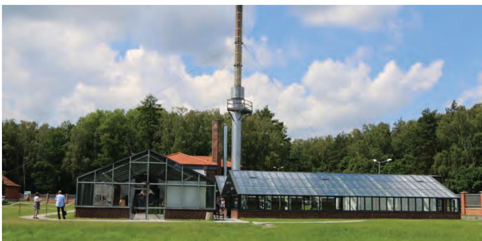
11. The exhibition rooms in the revitalised greenhouses
