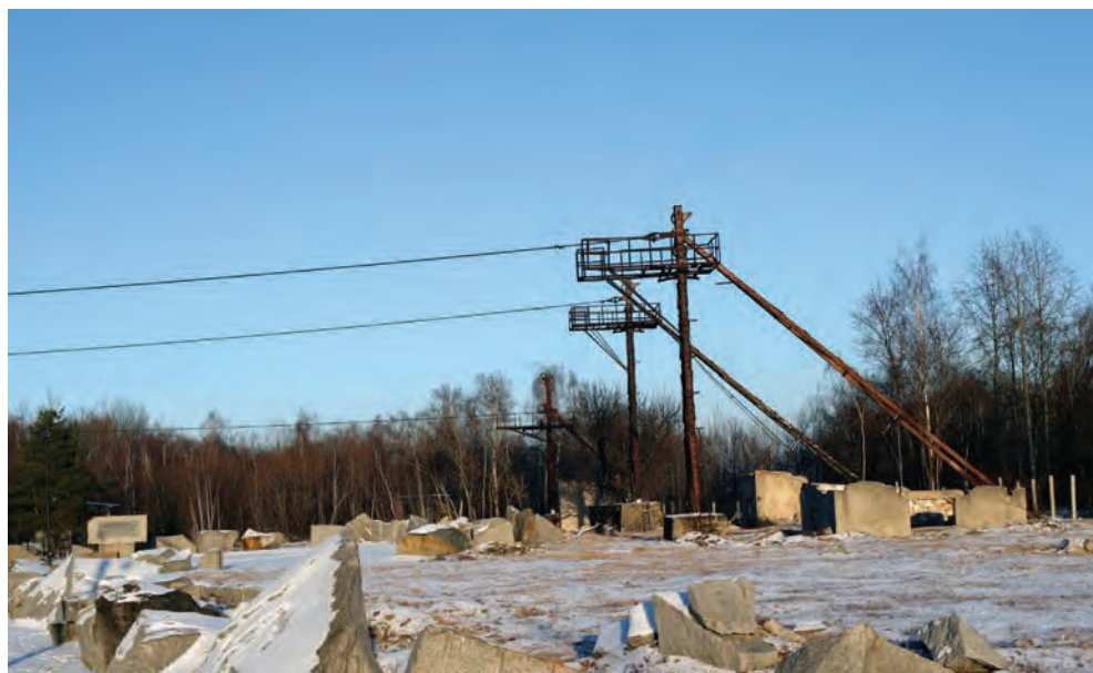
10. The historical mine infrastructure next to the quarry
