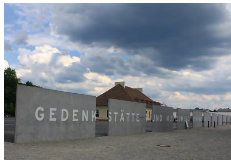
4. The entrance zone in front of the visitor centre building
