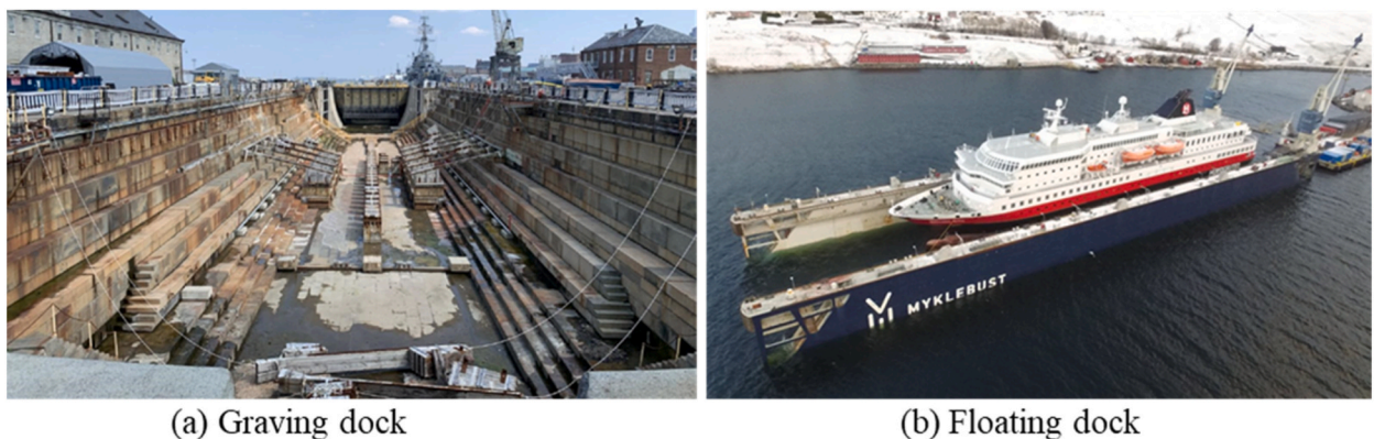
Fig. 1. Graving dock in Charlestown Navy Yard [3] and floating dock at Myklebust Verft AS [4].
