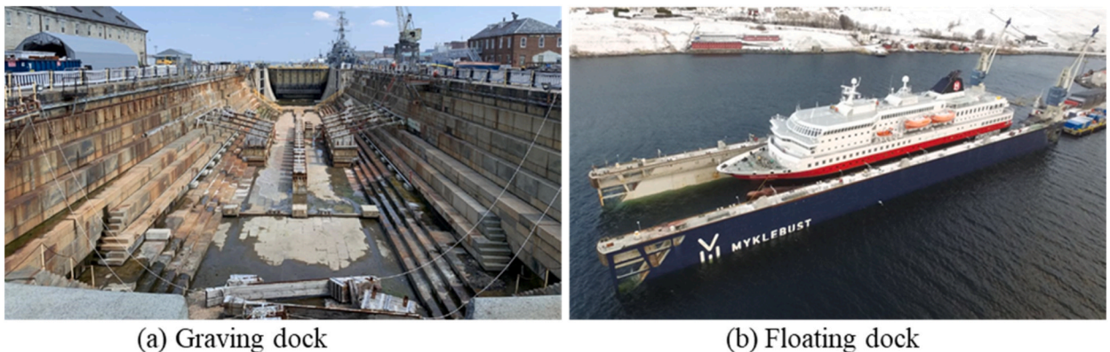
Fig. 1. Graving dock in Charlestown Navy Yard [3] and floating dock at Myklebust Verft AS [4].
