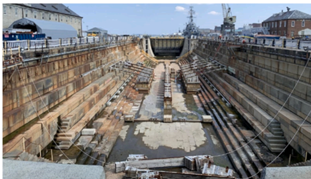
(a) Graving dock
