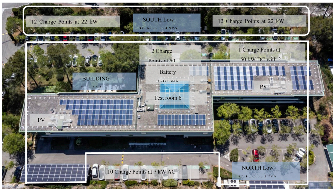
FIGURE 9 PV-driven setup of SAP France Labs (Kassem et al., 2023d).
