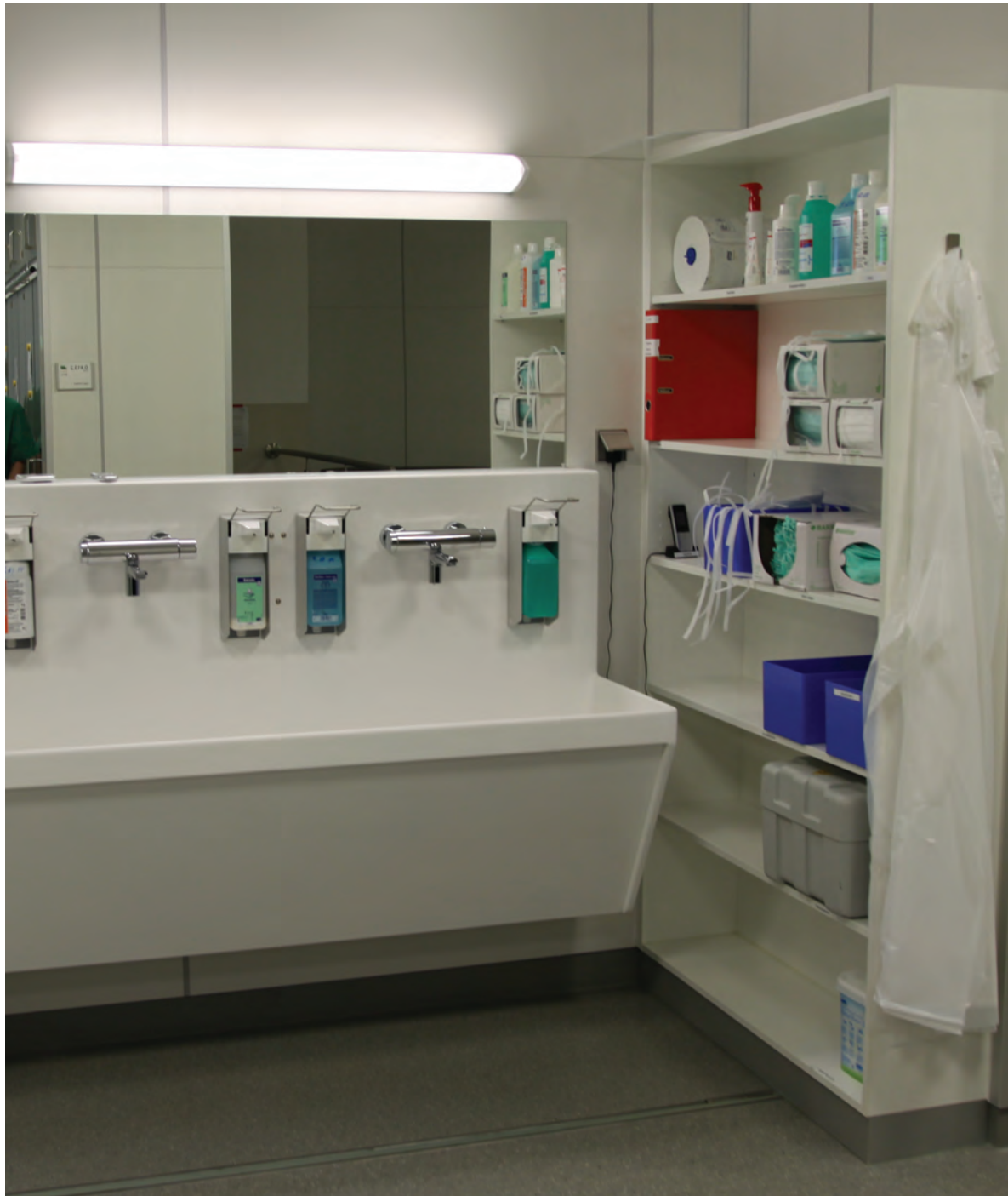
Photograph 4.1.2 A hand hygiene station in the operating suite circulation pathways (a solution excluded by the Polish legal regulations and applied in other countries); photographed by the Author, 2015
