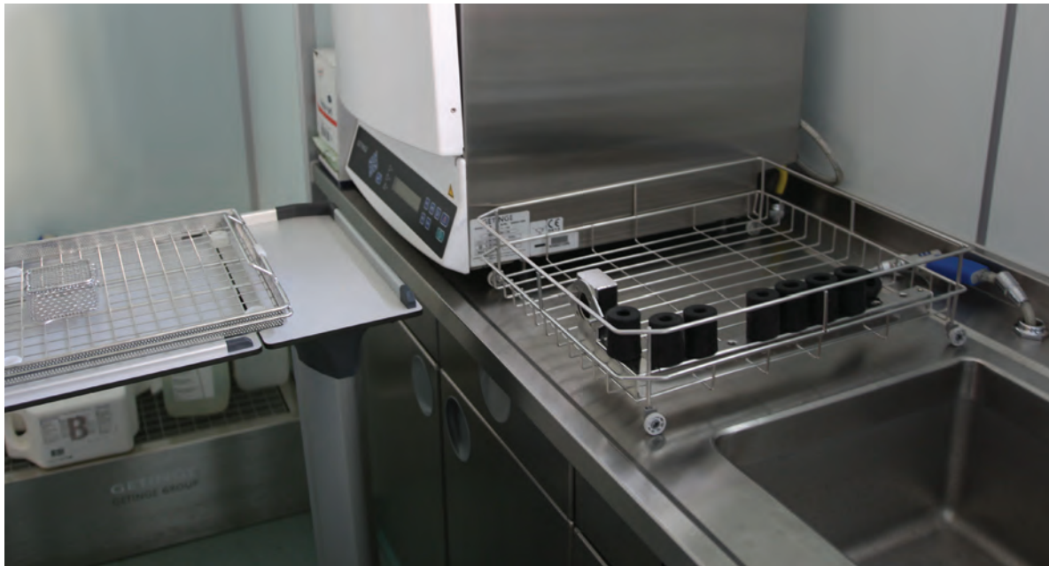
Photograph 5.4.3 A sterilisation unit (the progressive flow of materials is applied as a tool reducing contamination); photographed by the Author, 2016
