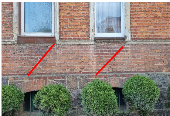
Fig. 4: Distribution of damages to the front wall (northern elevation) in the residential building: a) general view of the front elevation, b) left side (L) (basement part), c) right side (R) (non-basement part)
