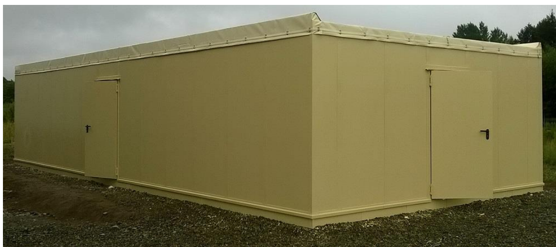
Figure 9. Prototype portable building constructed using modified composite sandwich panels
