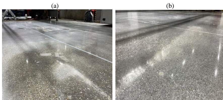
Fig. 8. Concrete industrial floor (Example 1) after repair: a) visible areas of repair of cavities b) visible areas of repair after anchors [38]
