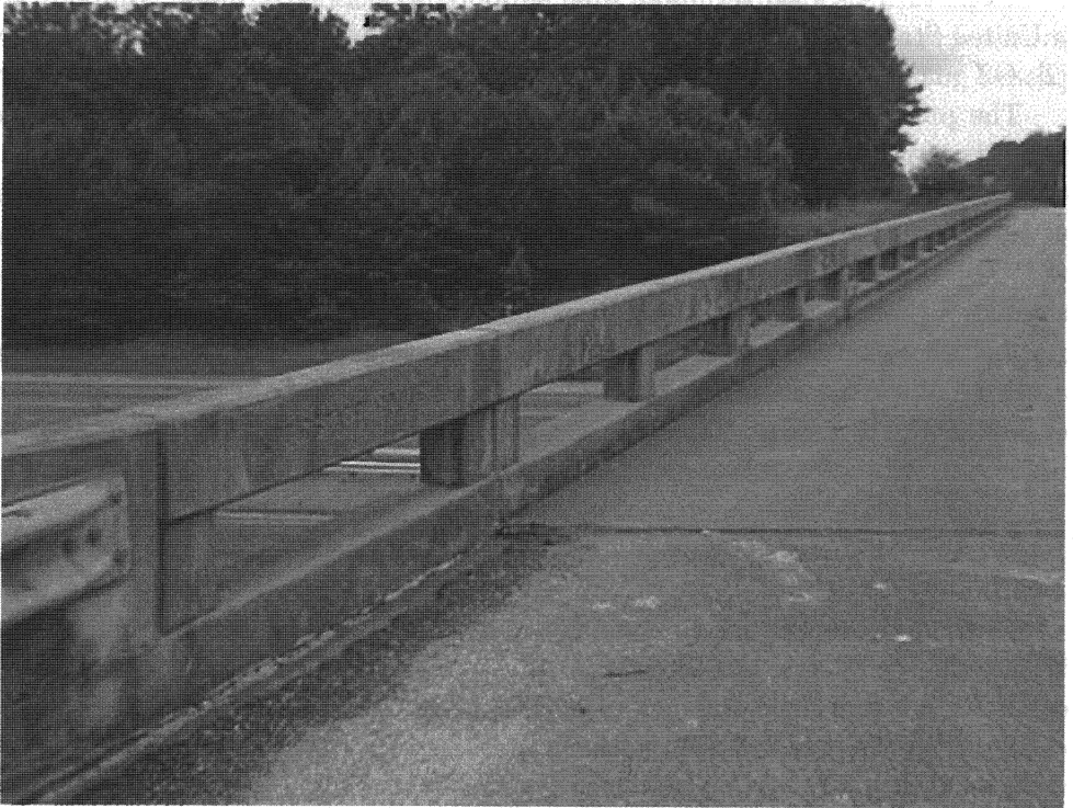
FIG. 1. An example of the Florida Beam-and-Post reinforced concrete bridge barrier (see text for description and dimensions).
