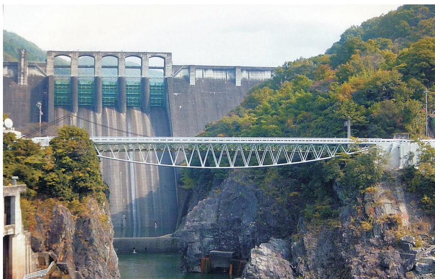
Rys.10. Most ukończony – widok boczny [7] Fig.10. Completed bridge – side view [7]
