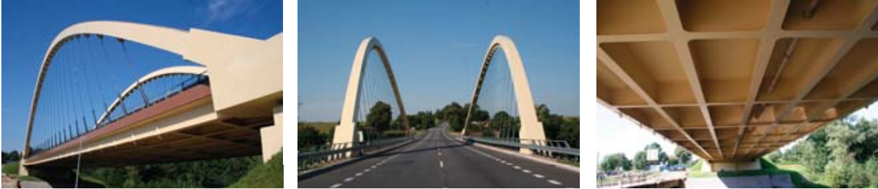
Fig. 3. Construction of the bridge in Poganice
