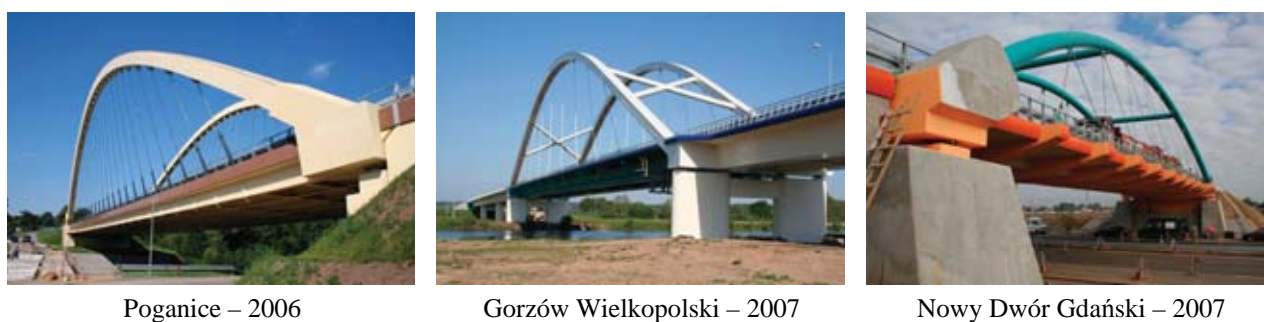
Fig. 2. Pictorial view of the analyzed overpasses
