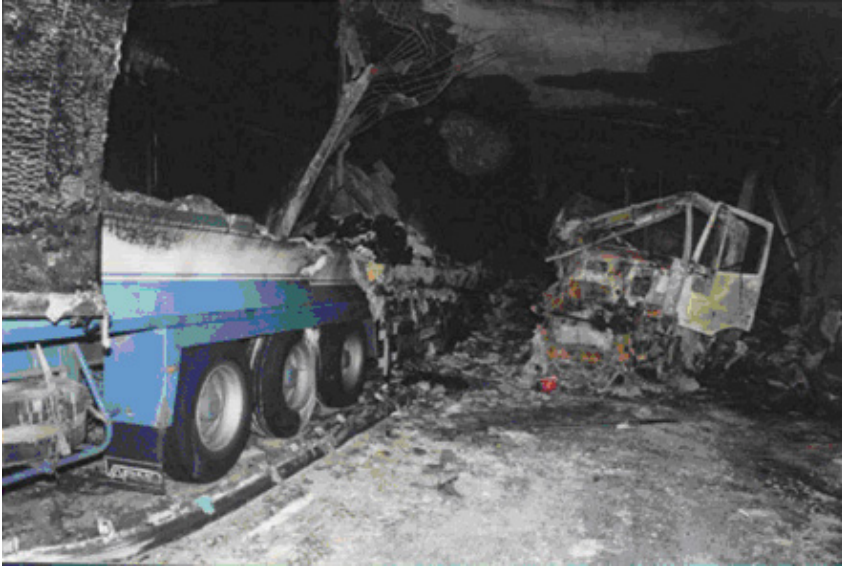
Fig. 1. The scene of accident in St. Gotthard road tunnel which was caused by a drunk driver [5]
