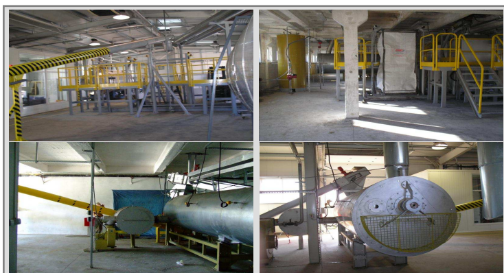
Fig. 3. Installation of BIOwęgiel® (biocarbon) production in Sedziszow (under construction) [6-8]
