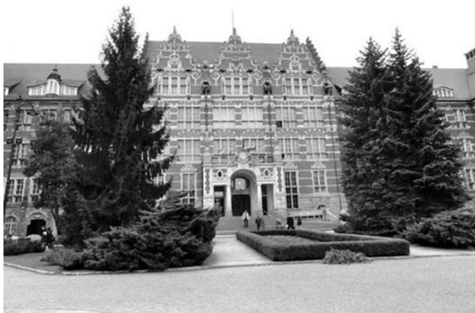
Fig. 17. The Main Building of the Technical University of Gdańsk ( Politechnika Gdańska ). Photograph by the author.
