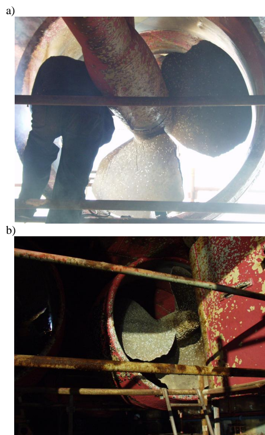
Fig. 6. Results of visual inspection of the propellers while the ship was put on the shipyard dock: a) damages of the port side propeller, b) damages of the starboard propeller
