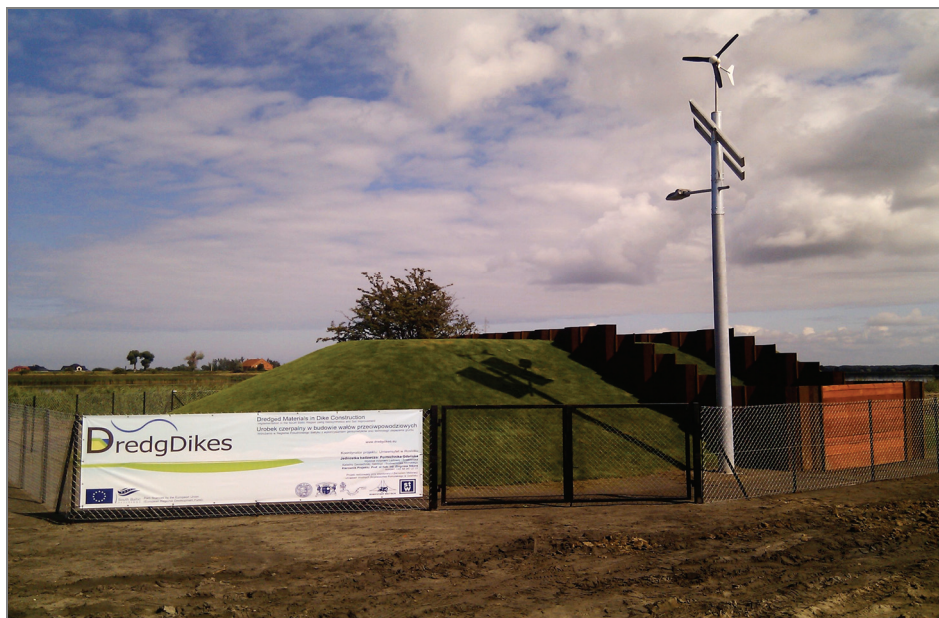
Fig. 1. View of the test dike
