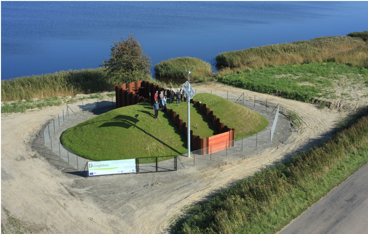
Fig. 1. The view of the experimental dike in Poland
