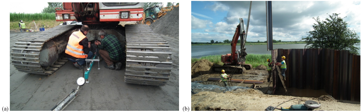
Fig. 5. Construction stages: (a) compaction verification – plate loading test (b) installation of sheet-pile wall
