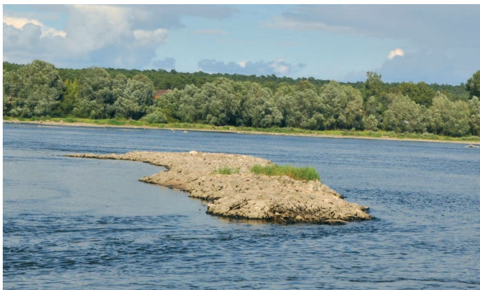
Photo 1. Groynes on the lower Vistula, photo: P. Jerzyło
