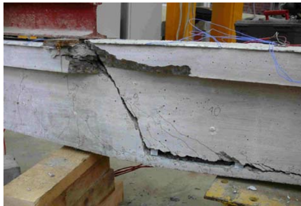
Fig. 7. Cracks in beam 1 on right hand side support
