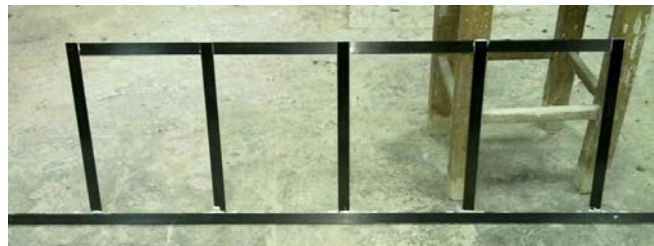
Fig. 3. Reinforcing cage before covering with sand
