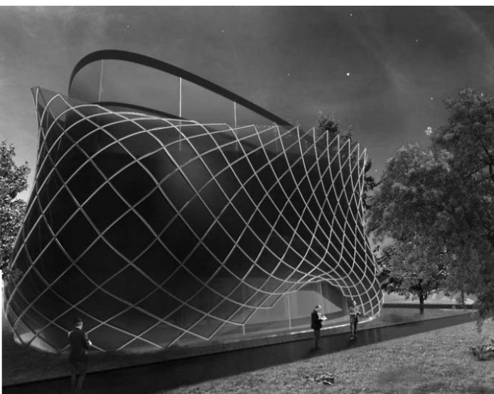
Fig. 4. Form+Facade, Office building, Zawadzki Lukas, Sopot College
