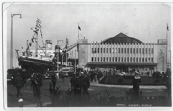
Fig. 1. The Gdynia Seaport Building, 1933 ( http://www.ronet.pl/ )
