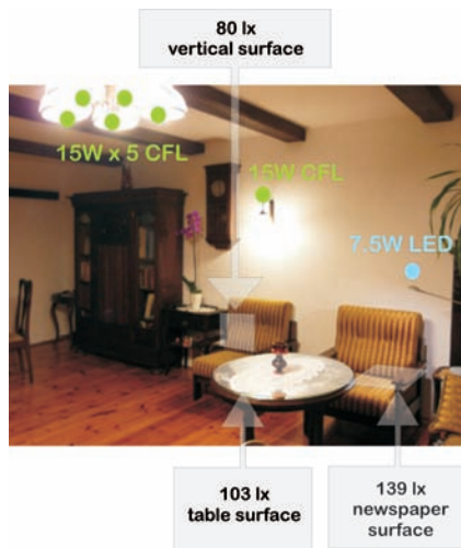
The new lighting for the reading task showing lux levels
