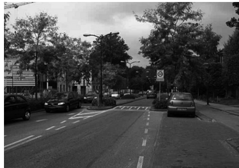
FIGURES 6 and 7. Natural barrier and entry to the 30 km per hour zone (K. Jamrozik, 2009)
