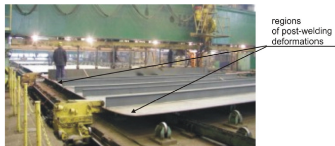
Fig. 1. Welding deformations of a plate section
