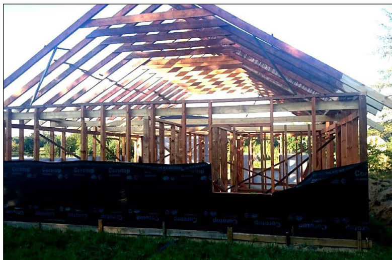
Fig. 1. Example of real size wooden house under construction
